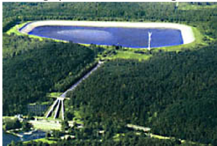
Pump storage Geesthacht near Hamburg
