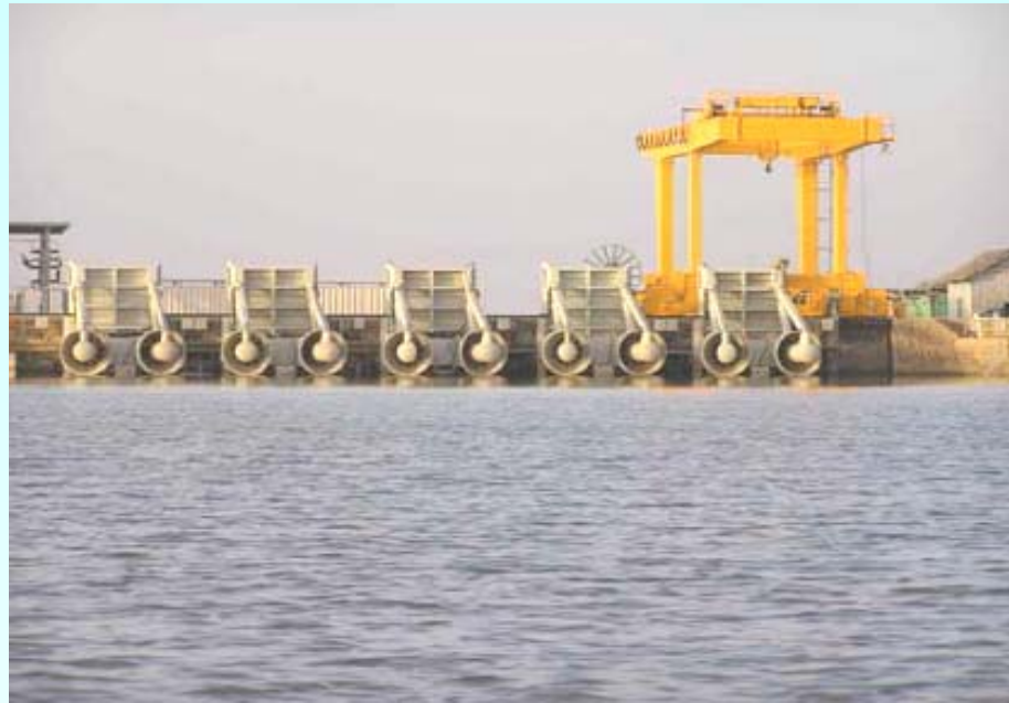
Power plant Djebel Aulia/Sudan-Nile
